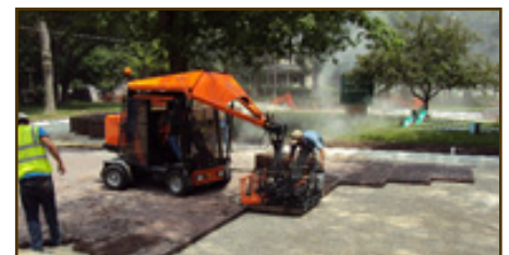
The largest permeable paving project in Iowa was completed in Charles City in 2010, eliminating localized flooding.
