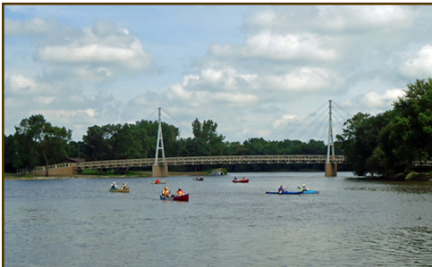
A group of flat-water river enthusiasts paddled under the new bridge and floated into the downtown area of Charles City for lunch.
